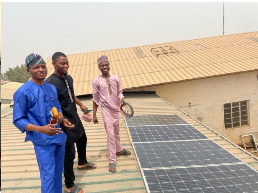
Figure 4.1b Installation of Solar Panel
