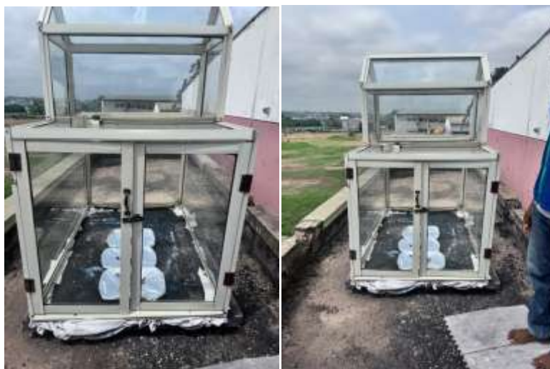
Figure 3.3.4 Complete construction of the greenhouse solar dryer
