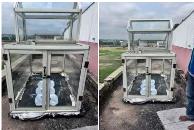
Figure 3.3.4 Complete construction of the greenhouse solar dryer
