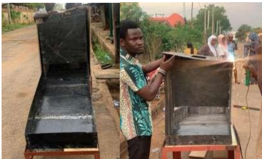
Figure 3.3.2 welded framework of the indirect solar dryer
