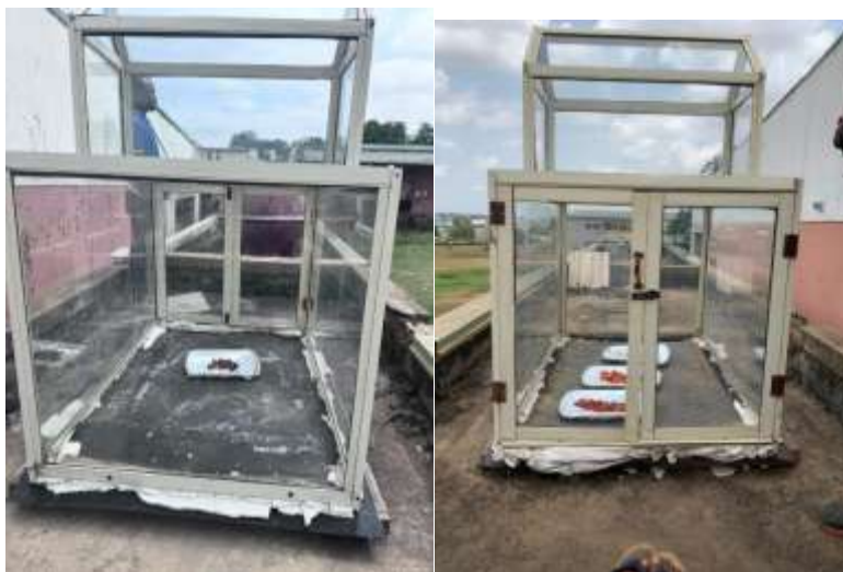
Figure 3.3.4 completed construction of the greenhouse solar dryer
