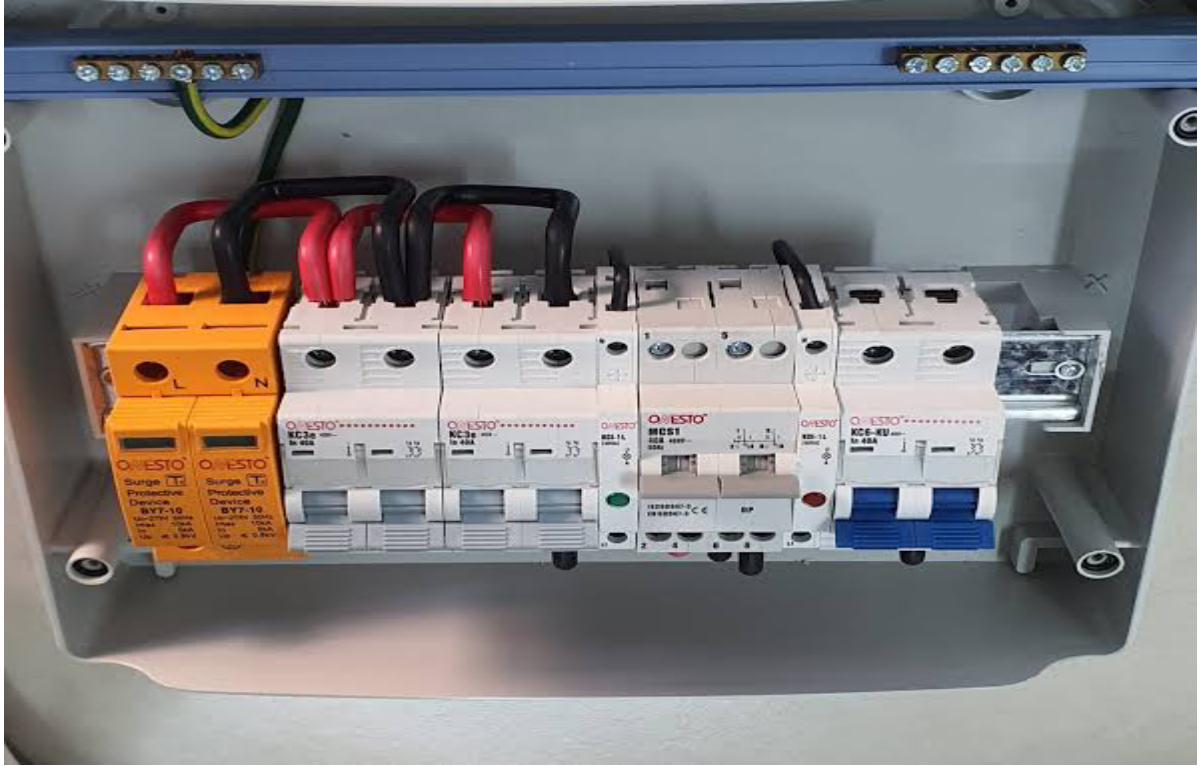
Figure 3.9: Protective Devices (Circuit breakers, SPD, Earthling)
