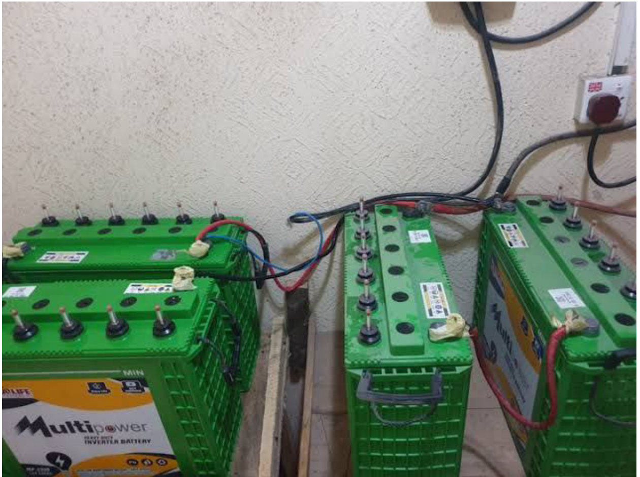
Figure 3.2: Battery Bank (Two Connected Batteries)
