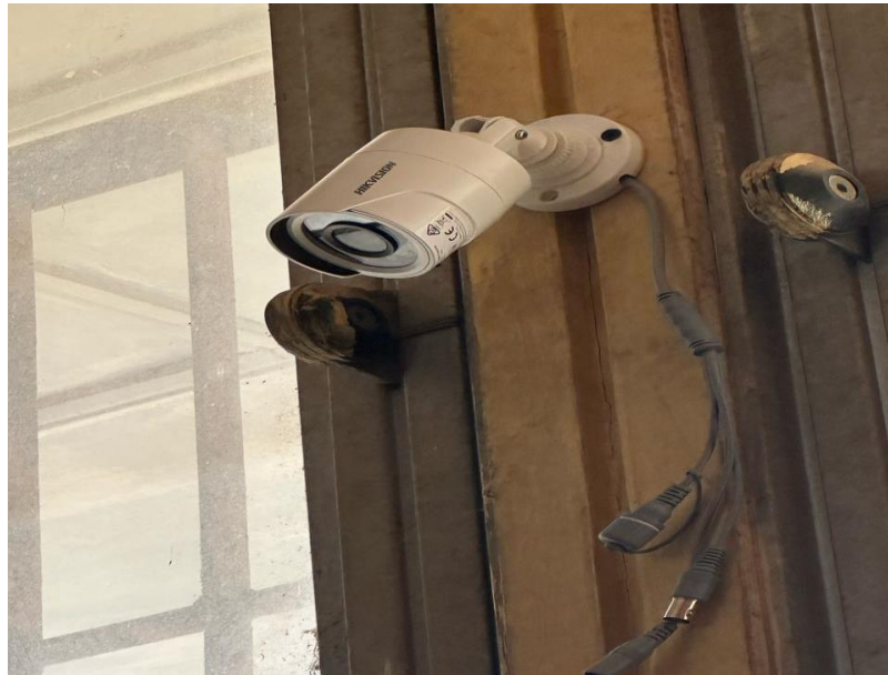
Fig 4.1.4: CCTV Camera Installation
