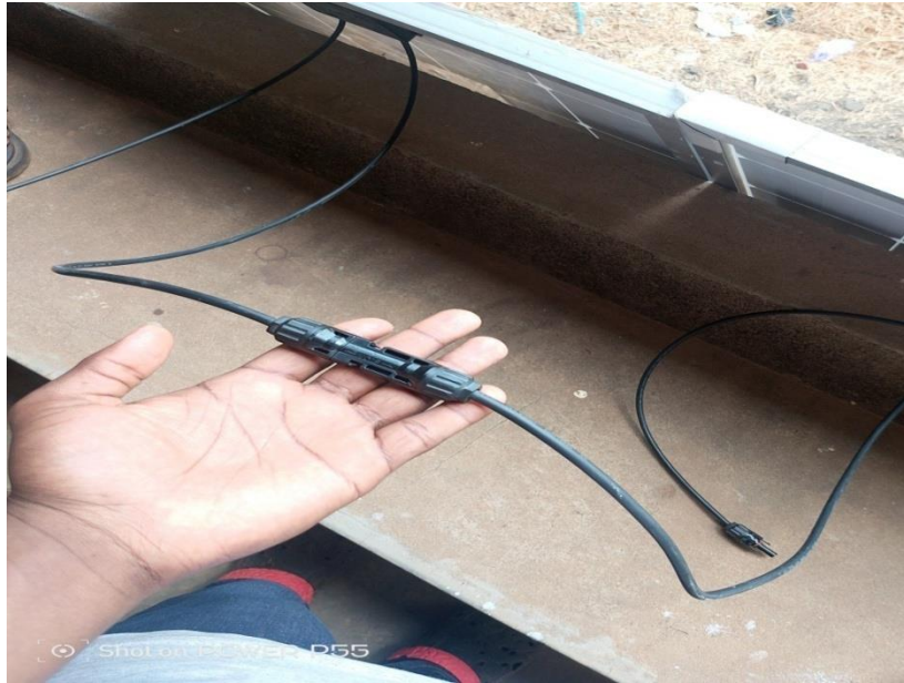
Fig 4.1.2 Solar panel installation (series from installation)
