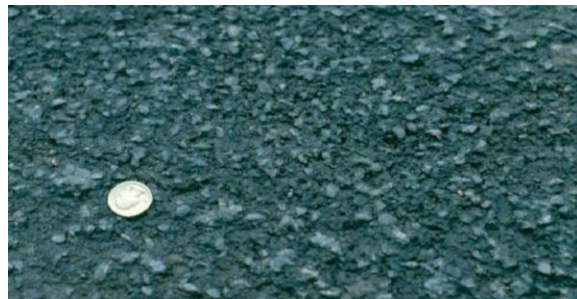
Fig: 7. High severity ravelling of asphalt surface
