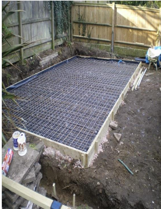
Fig 2.4: Mat (Raft) Foundation
