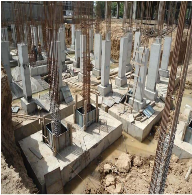
Fig. 2.1: Combined Footing Foundation
