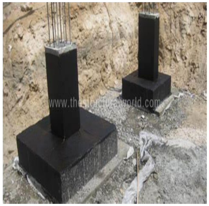
Fig. 2.2: Isolated Footing Foundation
