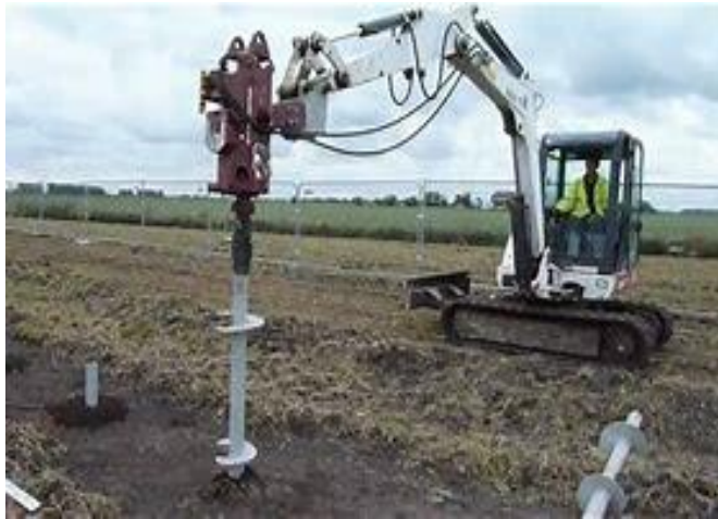
Fig. 2.8: Screw Piles Foundation
