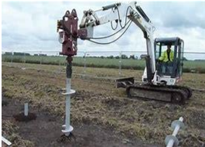
Fig. 2.8: Screw Piles Foundation
