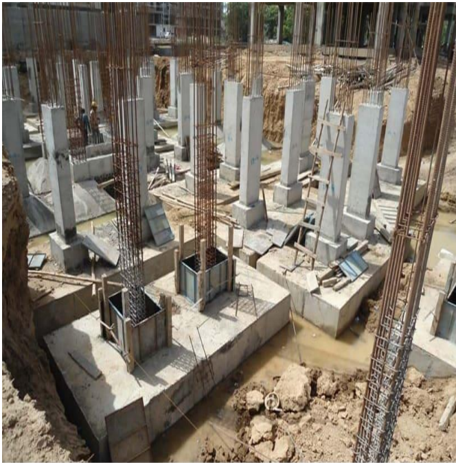
Fig. 2.1: Combined Footing Foundation
