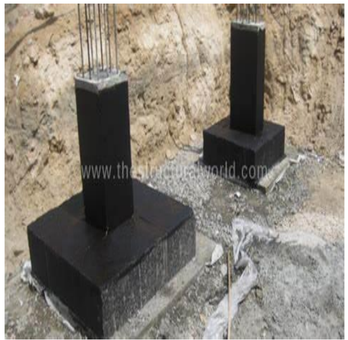
Fig. 2.2: Isolated Footing Foundation
