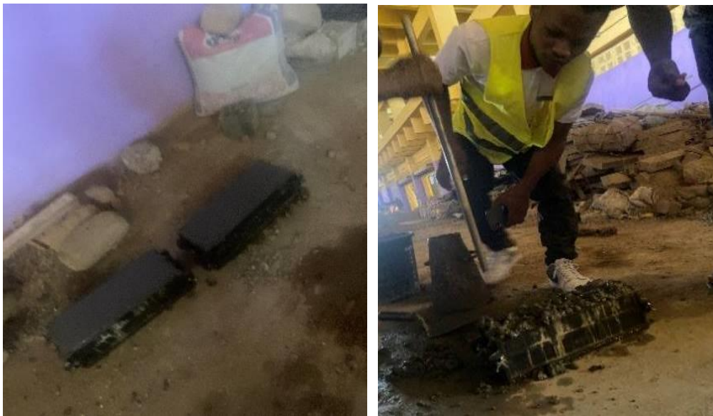
Figure 3.10: Casting of cubes
