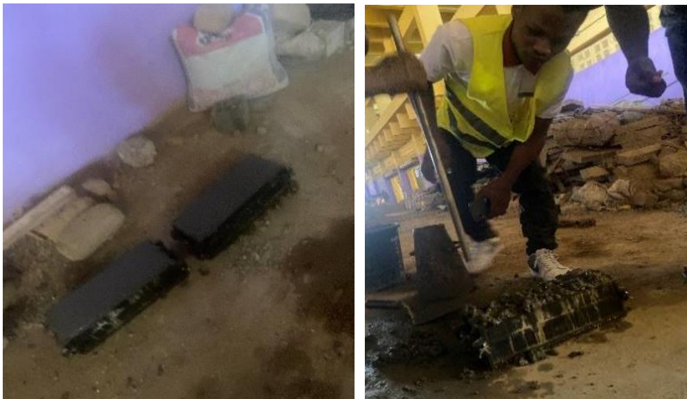
Figure 3.10: Casting of cubes
