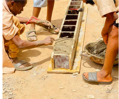
fig 3.5 : Casting of Specimen Cubes
