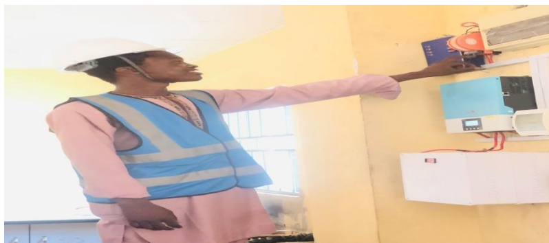
Figure 4.1d Complete Installation of Inverter with Lithium Battery
