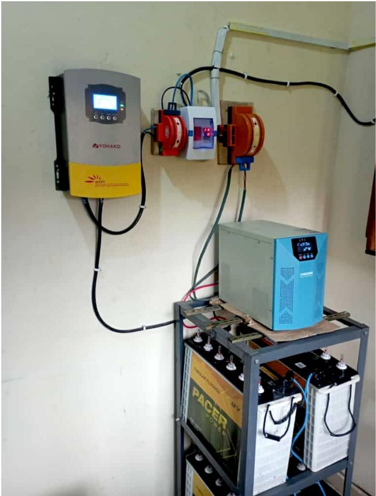
Fig. 3.6: Pictorial View of the 5KVA Hybrid Inverter System (Source Frank 2024)
