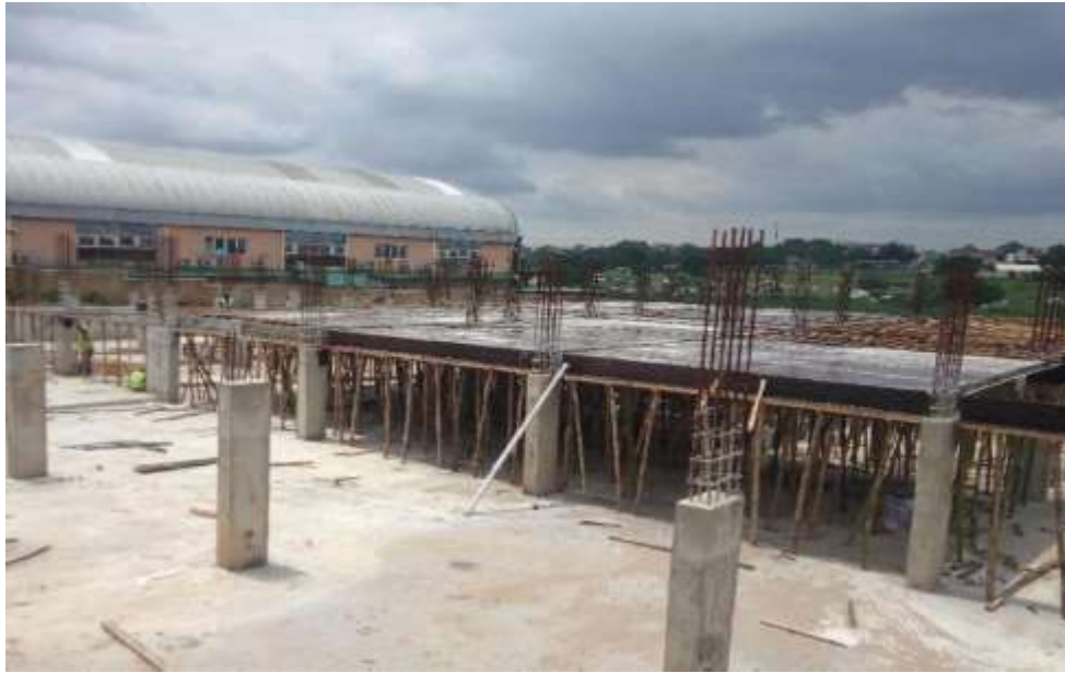
Plate 3.7: Form-work for the slab and beam.
