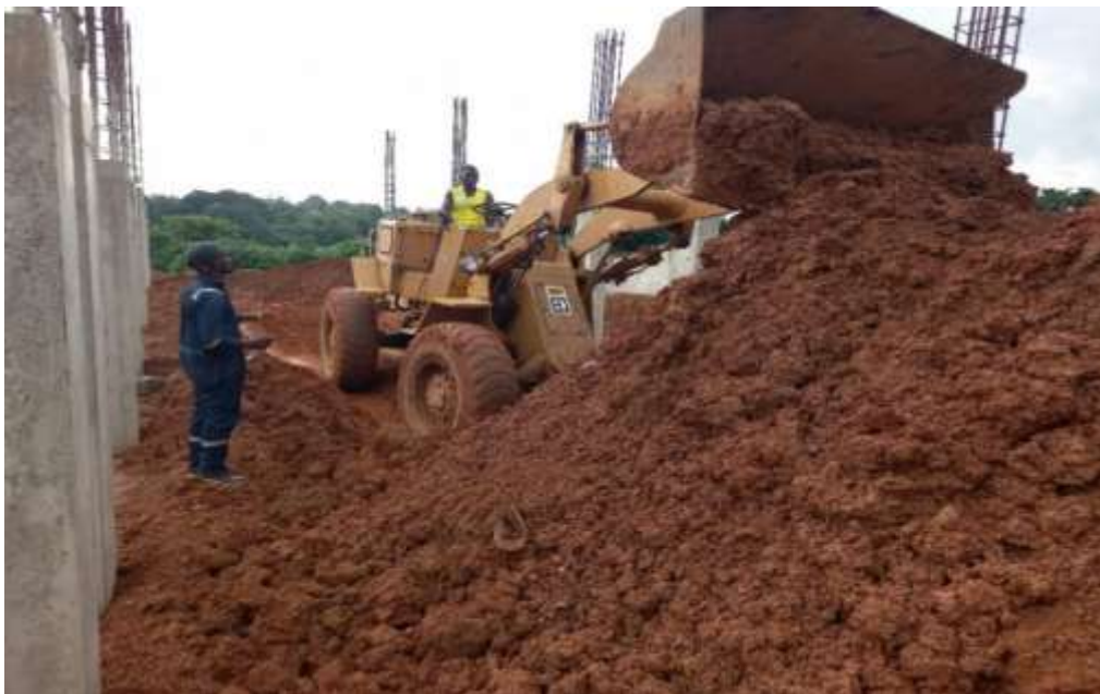
Backfilling of the basement using a front end loader.
