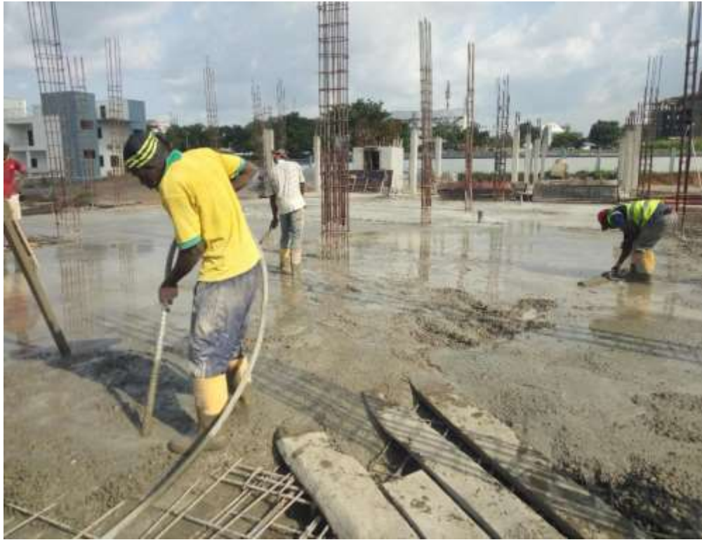
Plate 3.2: Showing Casting of slabs
