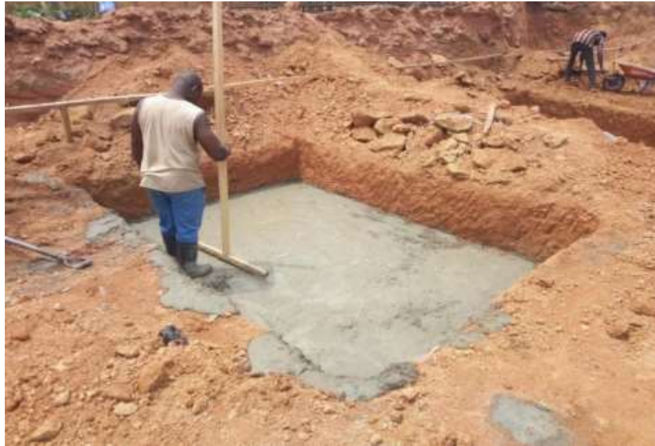
Plate 3.6: Blinding of the column-base(footing).
