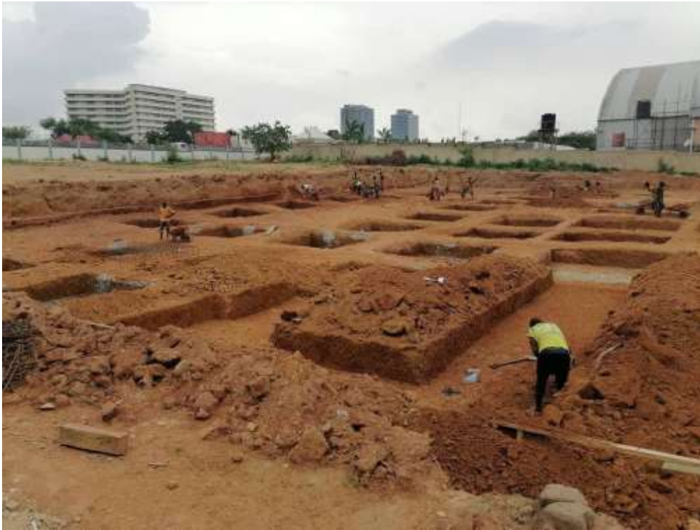
Plate 3.5: Excavating of the column base(footings) and foundation strips.
