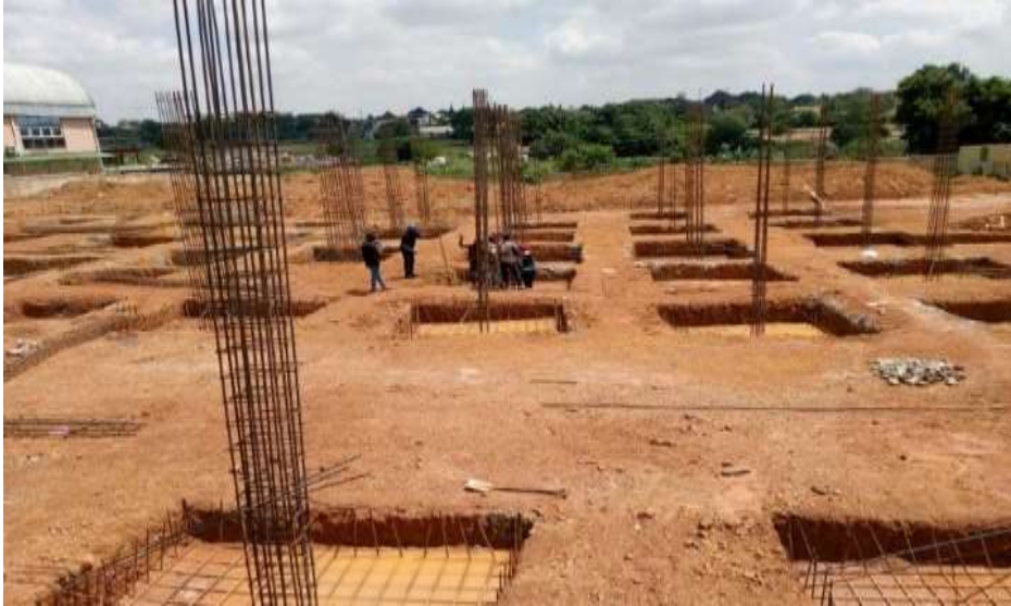
Plate 3.0: Showing Pad footings reinforcement works.
