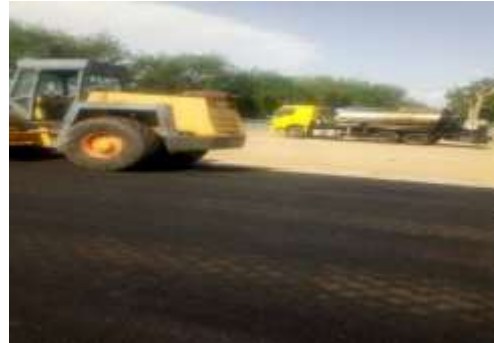
compaction of laid asphalt
