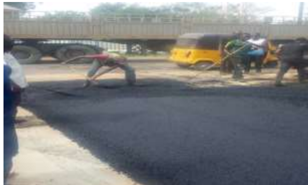
Workers spreading asphalt
