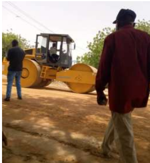
laterite compaction
