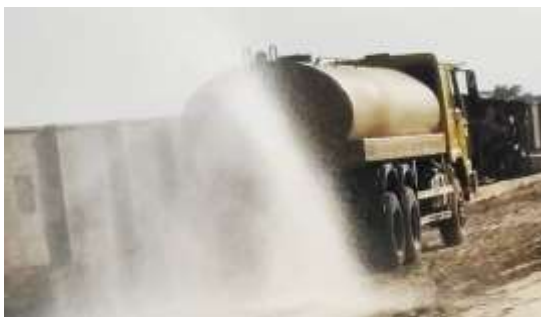
spraying of water by the water bauxer
