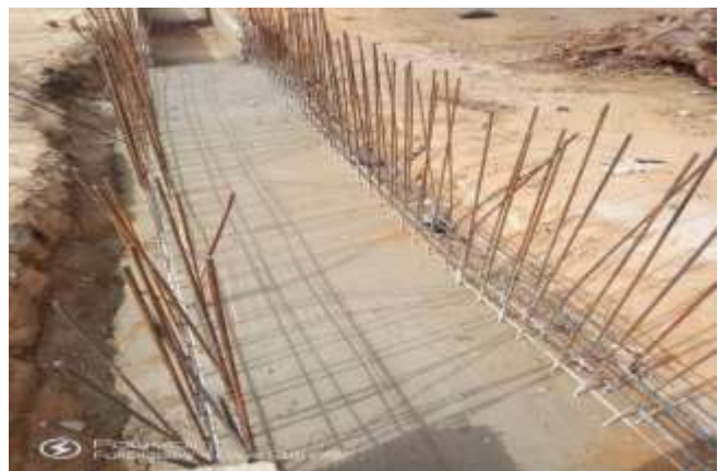
Arranged re-bars with concrete base
