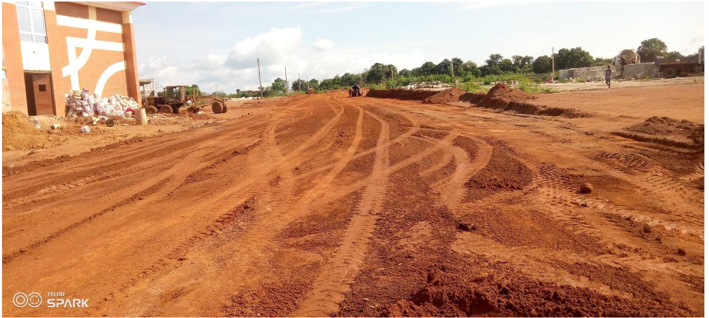
Grader scarifying and reshaping the roads for quality and drainage
