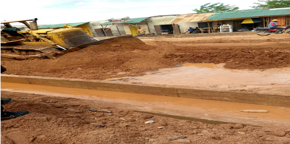
Figure 5.1: Heavy rainfall caused surface erosion and drainage blockage.
