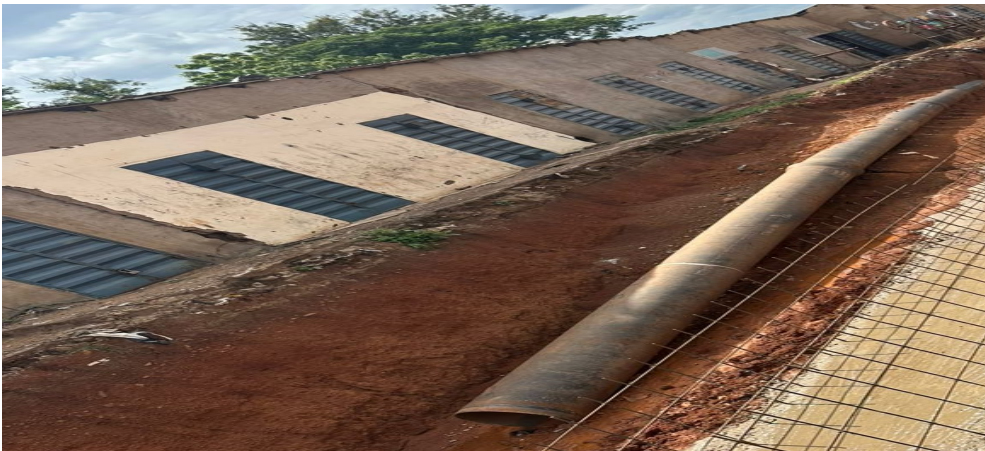
Figure 5.2: Transferring of water pipe in small length away from the drain line
