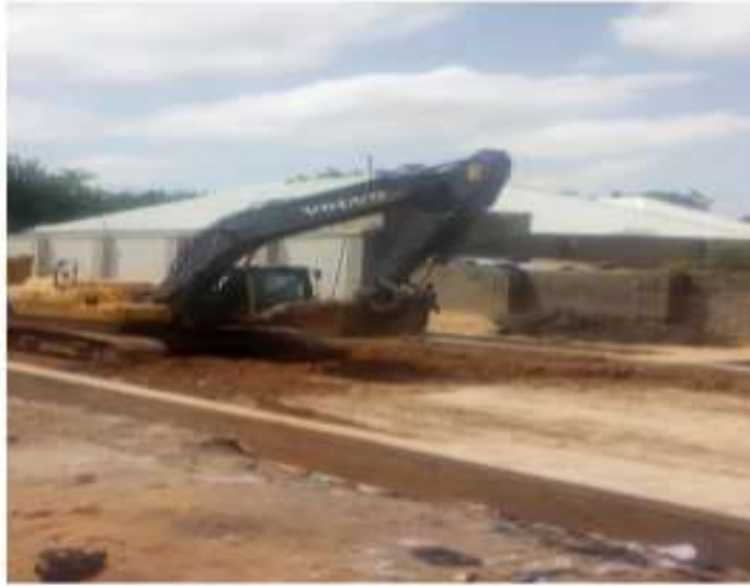
Plate 2.2: Roadway Excavation
