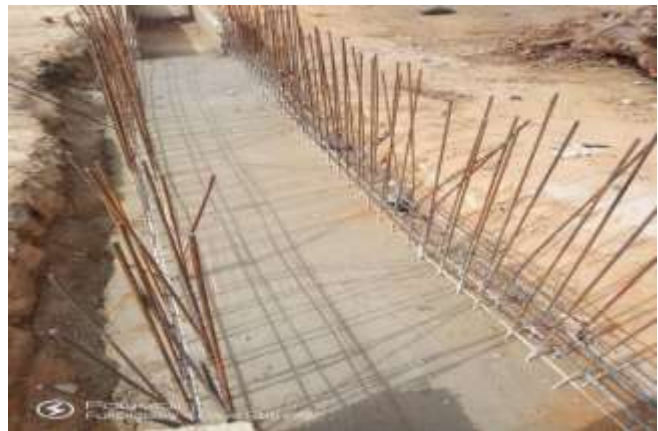
Arranged re-bars with concrete base
