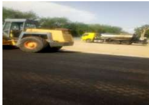
compaction of laid asphalt
