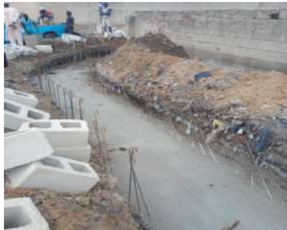
Blinding and concrete base
