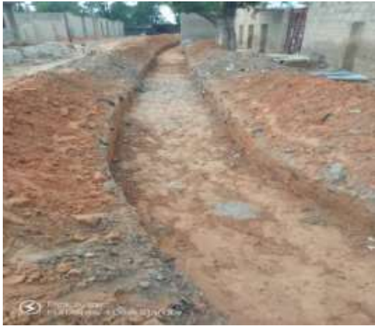
Excavated Drainage trench
