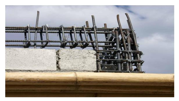
After the reinforcement then would be a framework which will be at the outer part of the reinforcement to guide the beam when casting.
