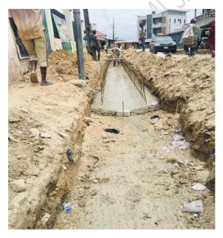
5. Construction of Formwork: this involves in propping and bracing of temporary structure known has formwork, which hold the concrete in place while it is set up for the construction of drainage wall.
