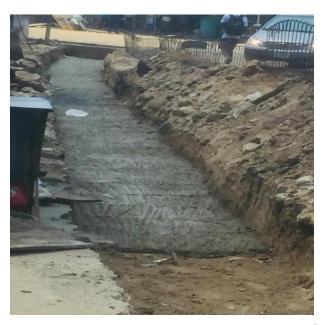
4. Fixing of Reinforcement and casting of concrete base: this is the process of pouring and shaping concrete to create the base for a drainage system. The concrete ratio use is 1:2:4
