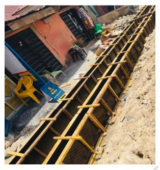
6. Casting off the drainage side walls: this involves pouring and shaping concrete to create vertical side wall for drainage structure. The concrete ratio use is 1:2:4
