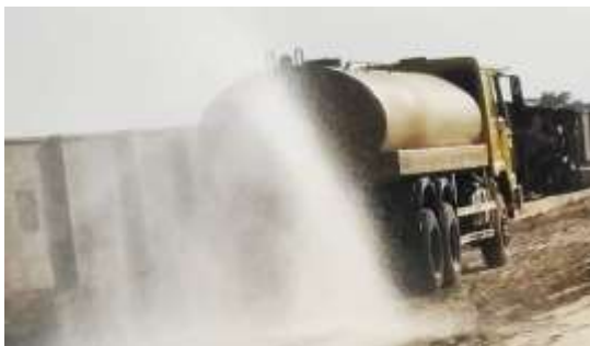
spraying of water by the water bauxer
