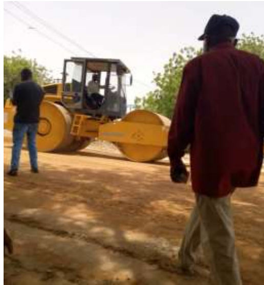
laterite compaction
