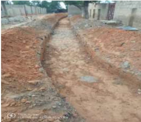
Excavated Drainage trench Plate
