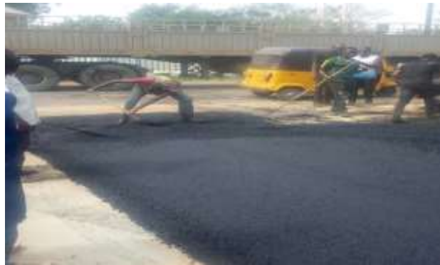
Workers spreading asphalt
