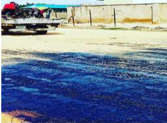
Blinding of the primed surface using quarry dust
