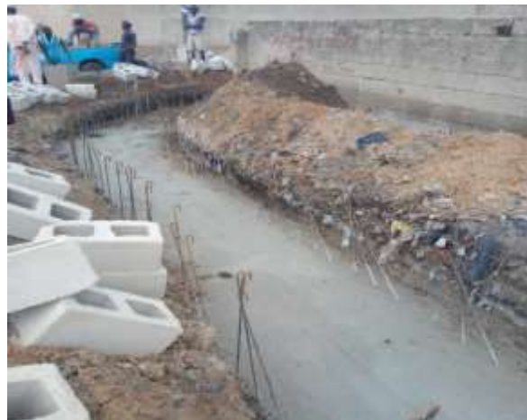
Blinding and concrete base
