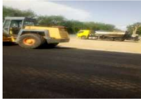
compaction of laid asphalt
