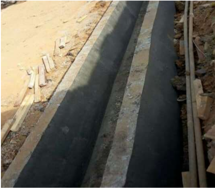
Drainage after casting
