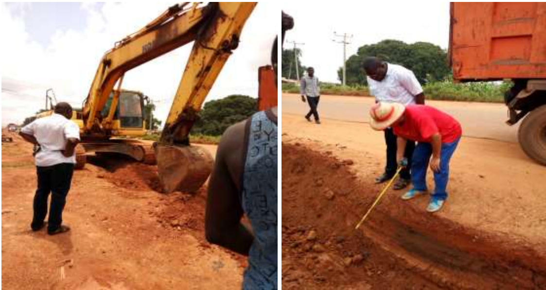
Fig4.2. Excavation of drainage trench with excavator machine
