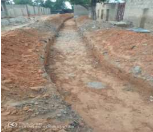
Excavated Drainage trench Plate
