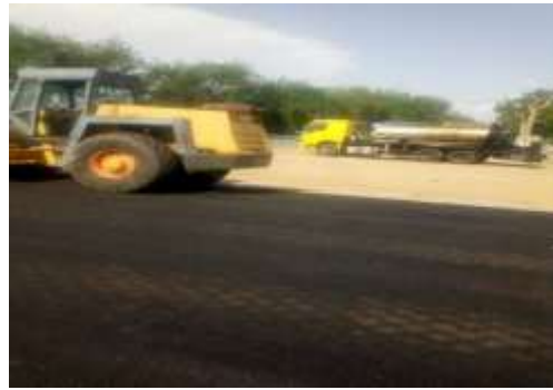
compaction of laid asphalt
