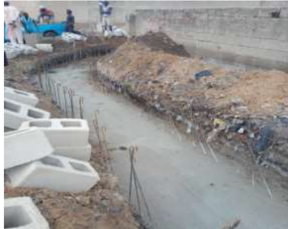
Blinding and concrete base
