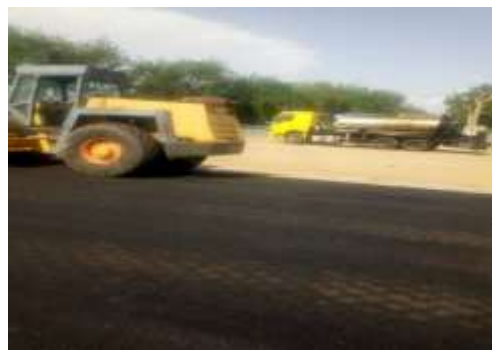
compaction of laid asphalt
