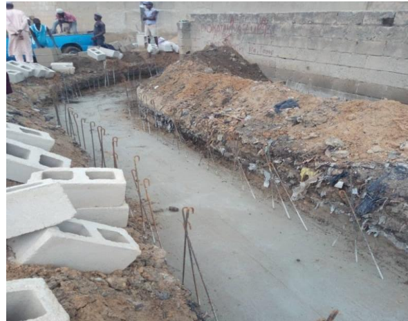
Blinding and concrete base
