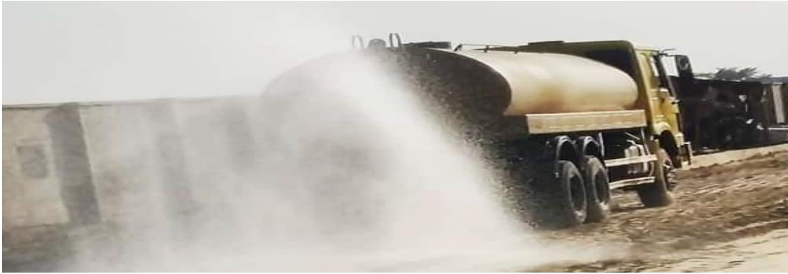
spraying of water by the water bauxer
