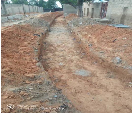
Excavated Drainage trench Plate
