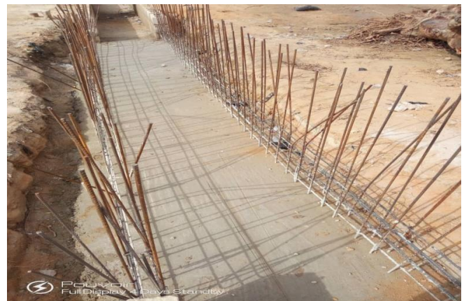
Arranged re-bars with concrete base
