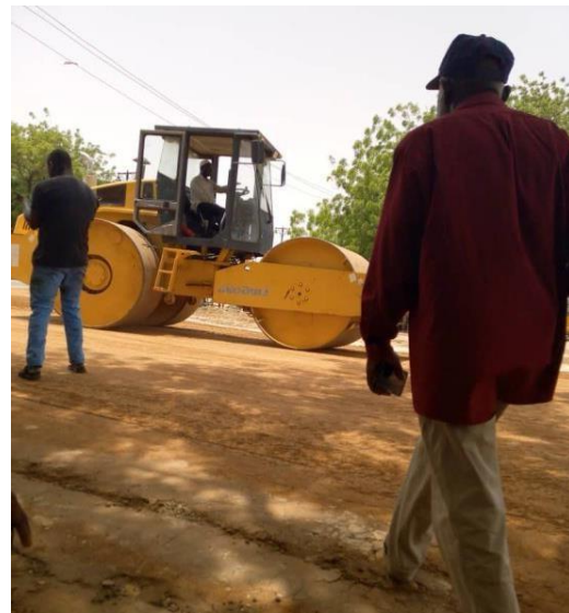
laterite compaction
