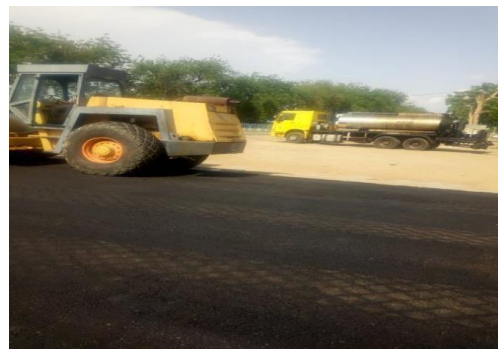
compaction of laid asphalt
