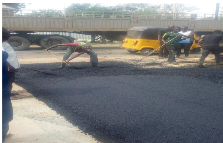
Workers spreading asphalt
