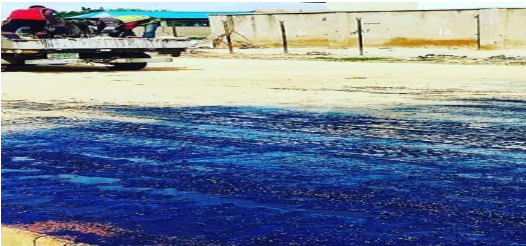
Blinding of the primed surface using quarry dust
