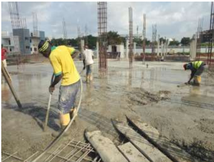
Showing Casting of slabs
