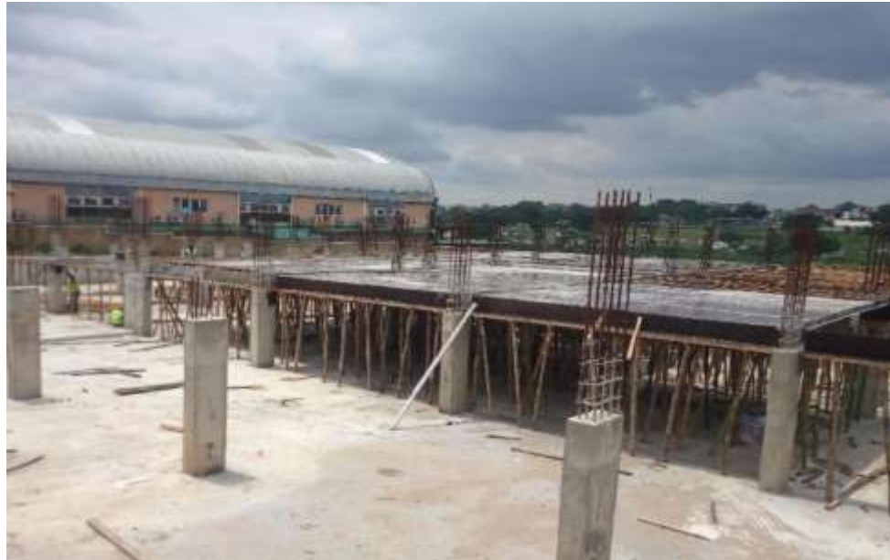
Plate 3.7: Form-work for the slab and beam.
