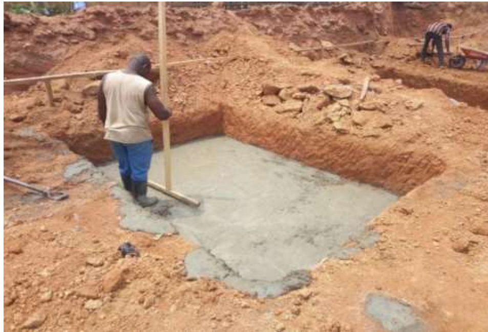
Plate 3.6: Blinding of the column-base(footing).
