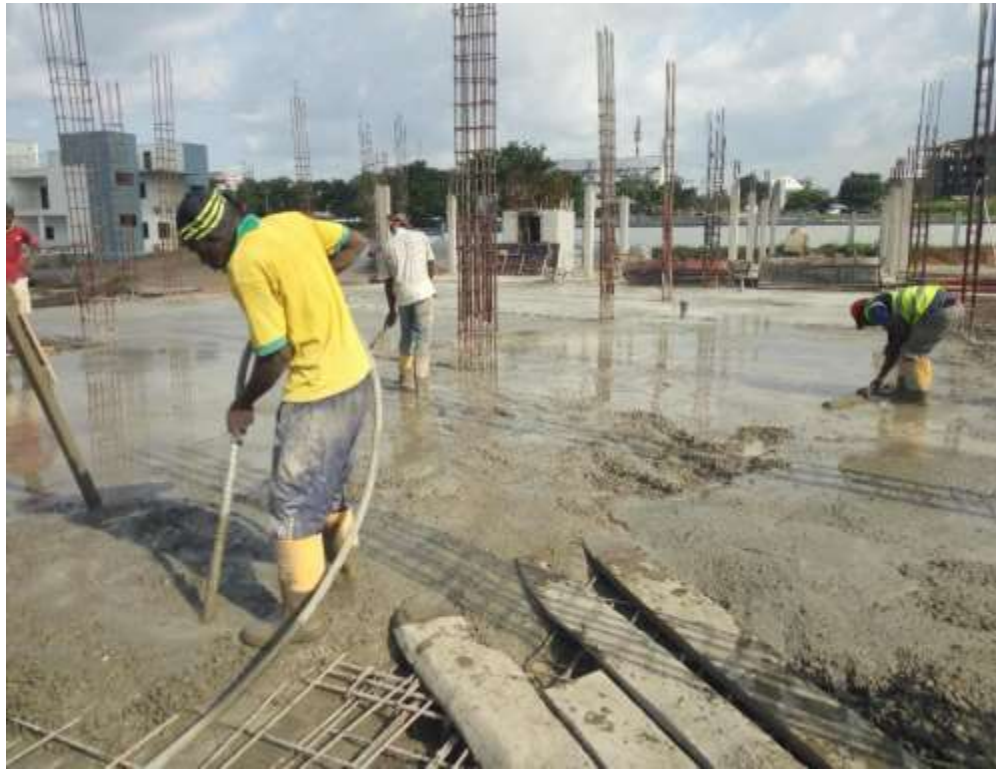
Plate 3.2: Showing Casting of slabs
