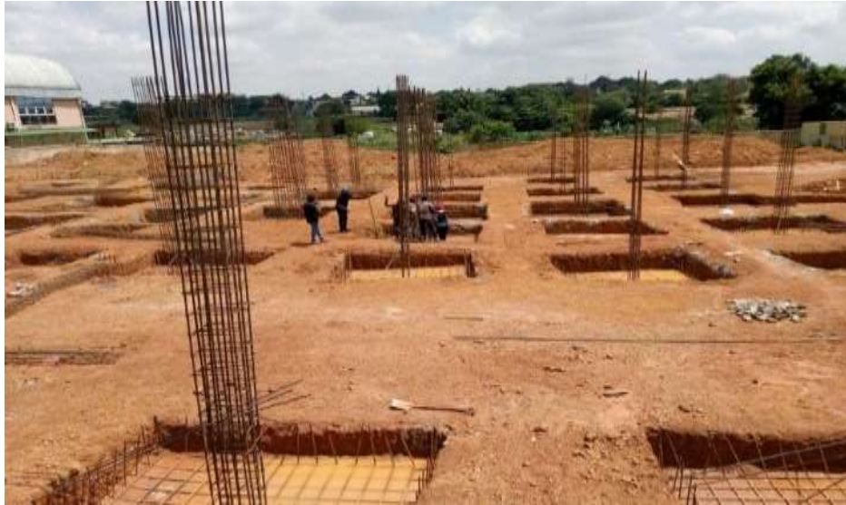
Plate 3.0: Showing Pad footings reinforcement works.
