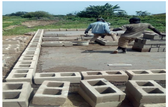
Image 9: showing block forming after DPC
