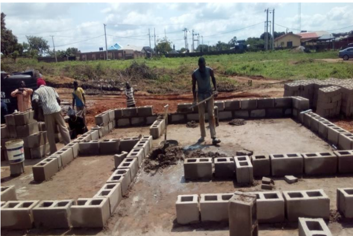
Image 10: showing block forming after DPC
