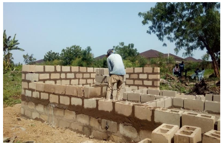
Image 9: showing block work in superstructure
