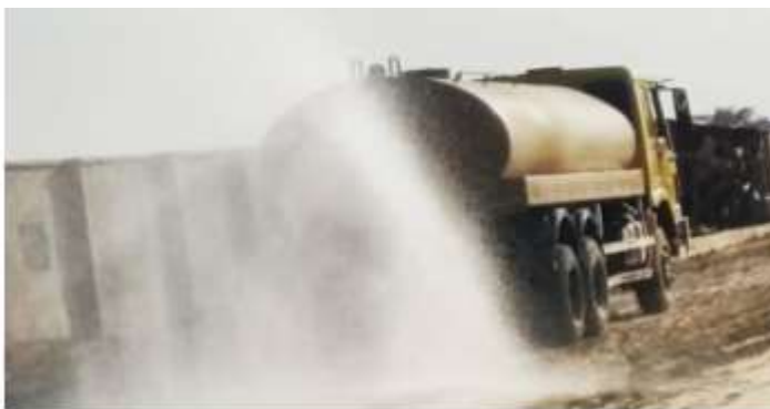
spraying of water by the water bauxer
