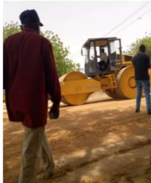
laterite compaction
