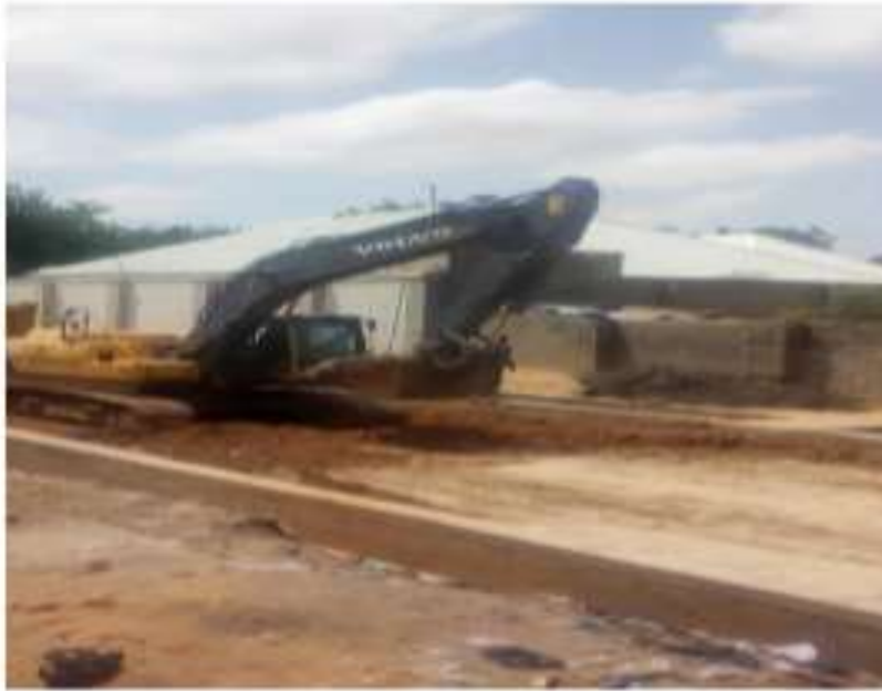
Plate 2.2: Roadway Excavation
