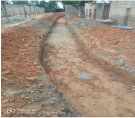
Plate 4.0: Excavated Drainage trench
