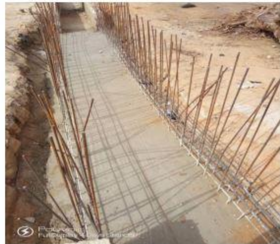
Plate 4.3: Arranged re-bars with concrete base
