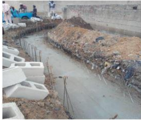
Plate 4.1: Blinding and concrete base
