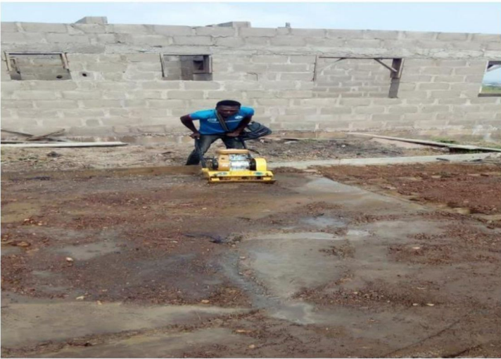
Image 2: showing compaction of soil by manual compacting machine
