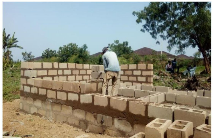
Image 4: showing block work in superstructure
