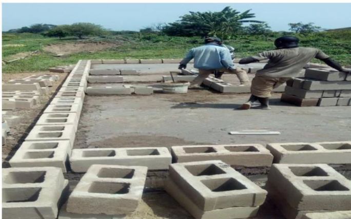
Image 3: showing block forming after DPC
