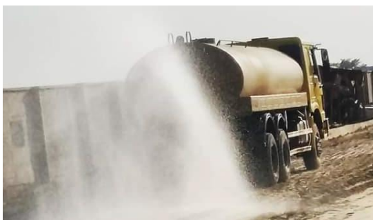
spraying of water by the water bauxer
