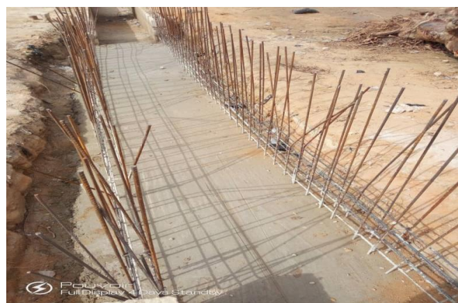
Arranged re-bars with concrete base
