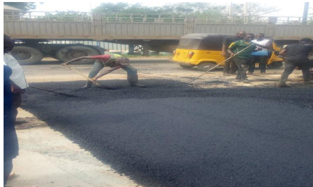
Workers spreading asphalt
