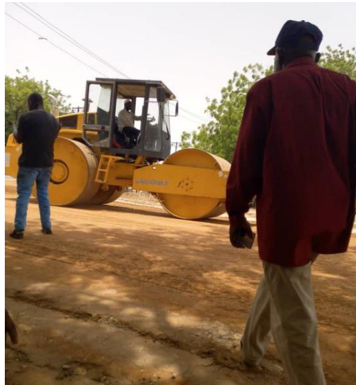
laterite compaction
