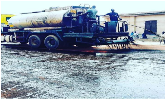
Bitumen Boiler
