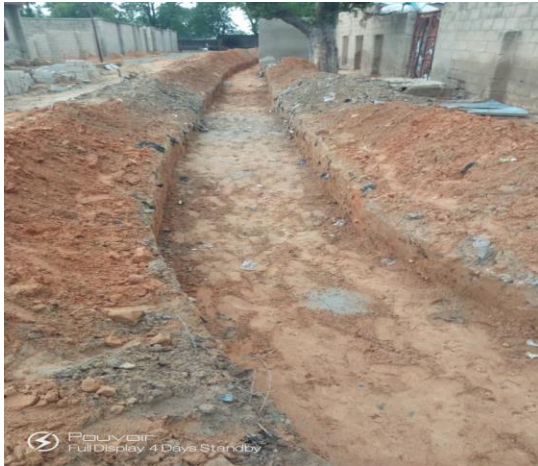
Excavated Drainage trench Plate
