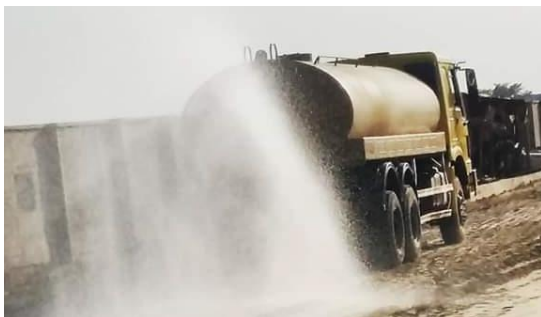
spraying of water by the water bauxer
