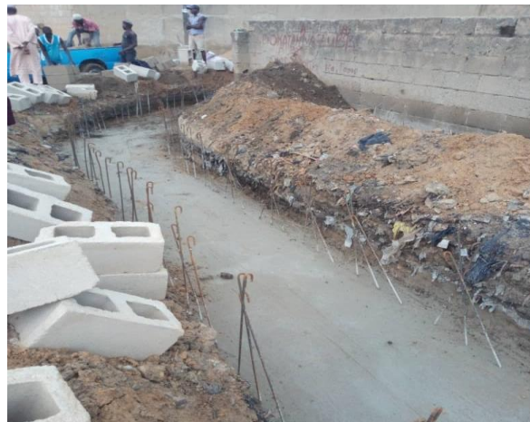
Blinding and concrete base
