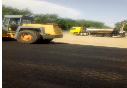
compaction of laid asphalt
