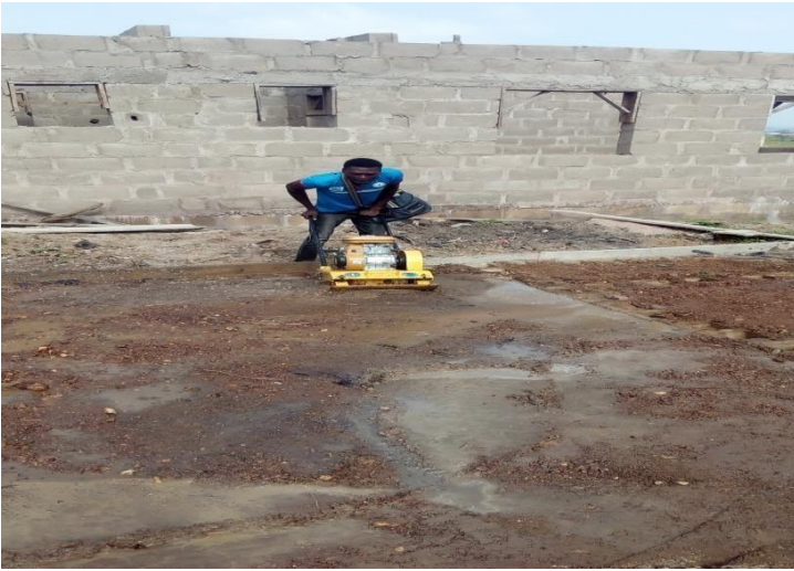
Image 6: showing compaction of soil by manual compacting machine
