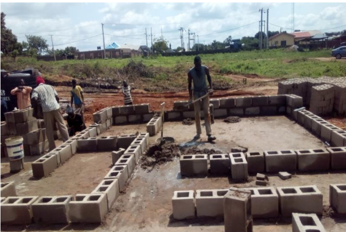
Image 10: showing block forming after DPC
