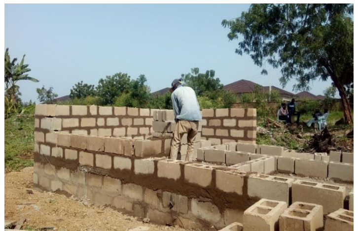
Image 9: showing block work in superstructure
