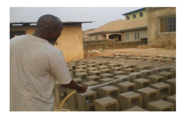
FIGURE THREE: PICTORIAL VIEW OF WETING OFBRICK BLOCKS
