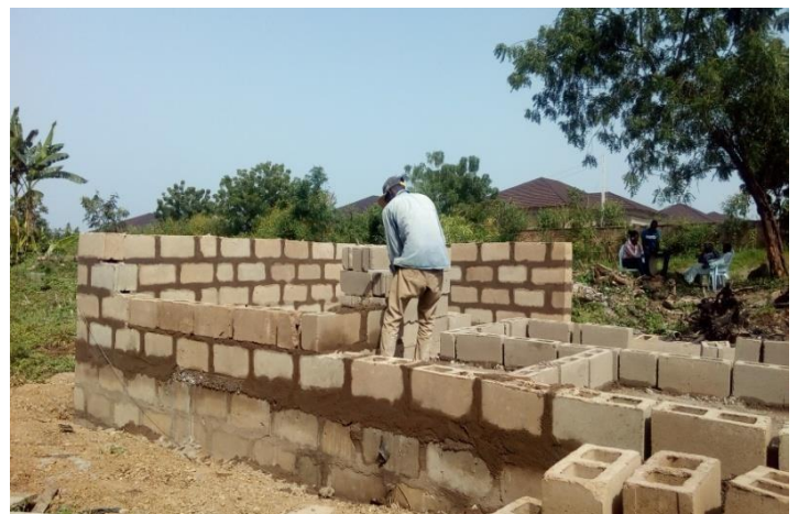
Image 9: showing block work in superstructure
