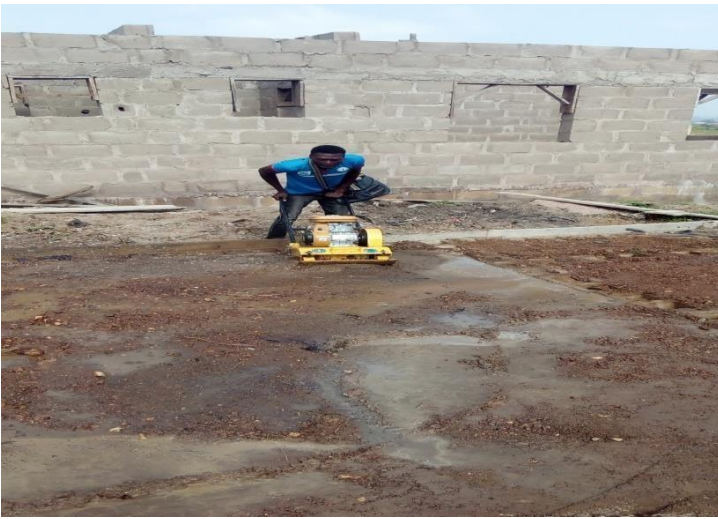
Image 6: showing compaction of soil by manual compacting machine
