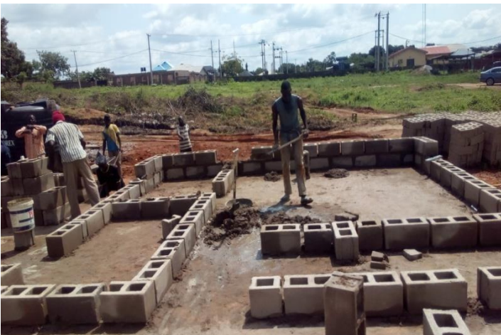
Image 10: showing block forming after DPC
