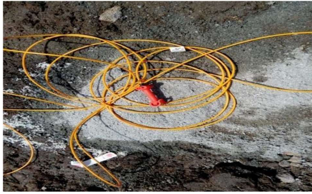
Figure 3.5c: Non-electric detonator
