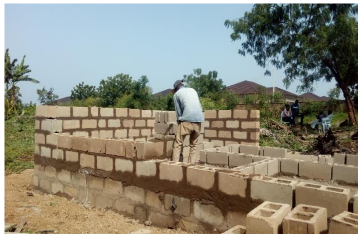
Image 9: showing block work in superstructure
