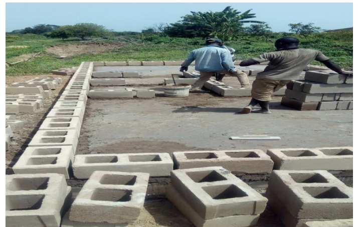
Image 9: showing block forming after DPC
