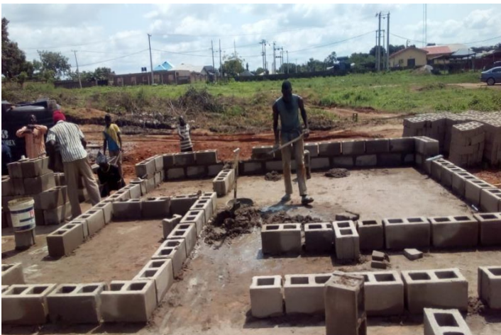
Image 10: showing block forming after DPC
