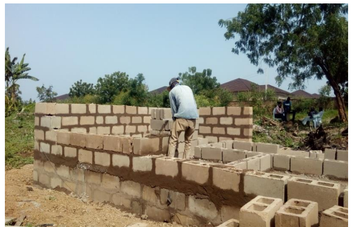
Image 9: showing block work in superstructure
