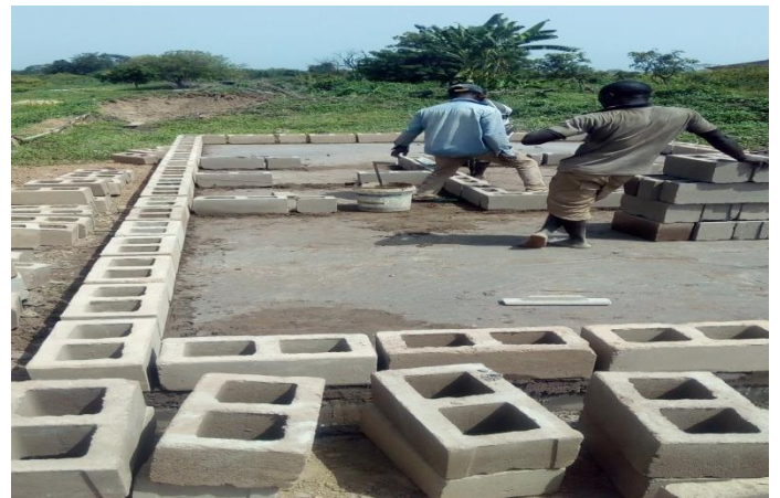
Image 9: showing block forming after DPC
