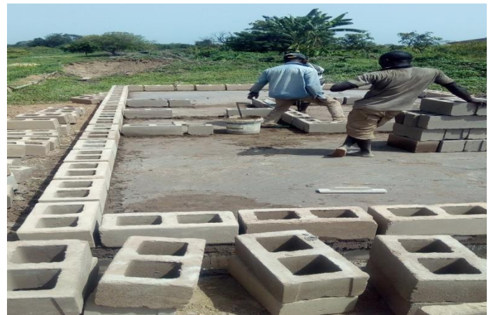
Image 9: showing block forming after DPC
