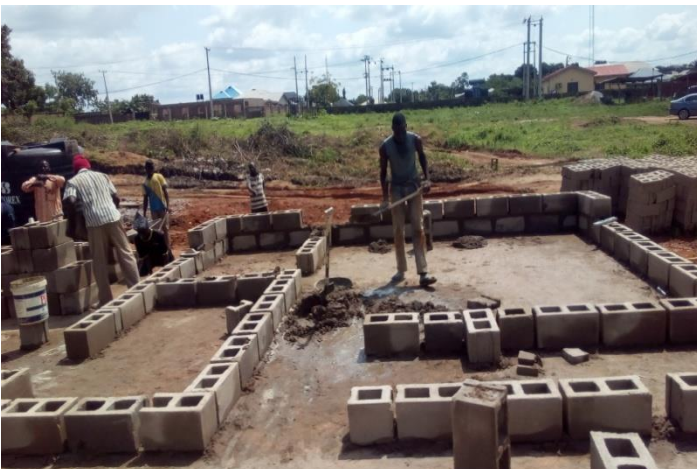
Image 10: showing block forming after DPC
