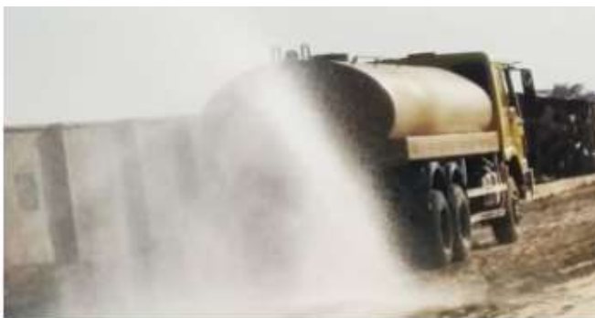
spraying of water by the water bauxer
