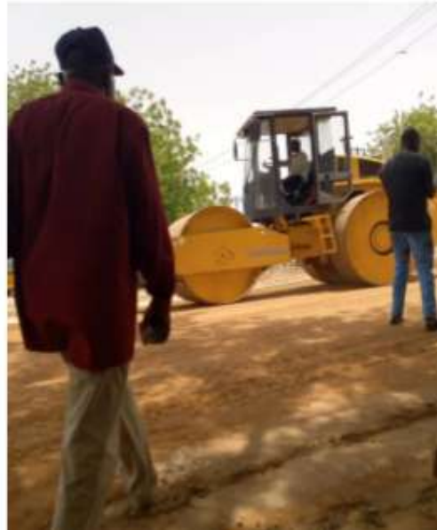
laterite compaction
