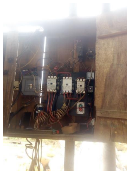
Fig. 3: Installed Star-Delta starter
