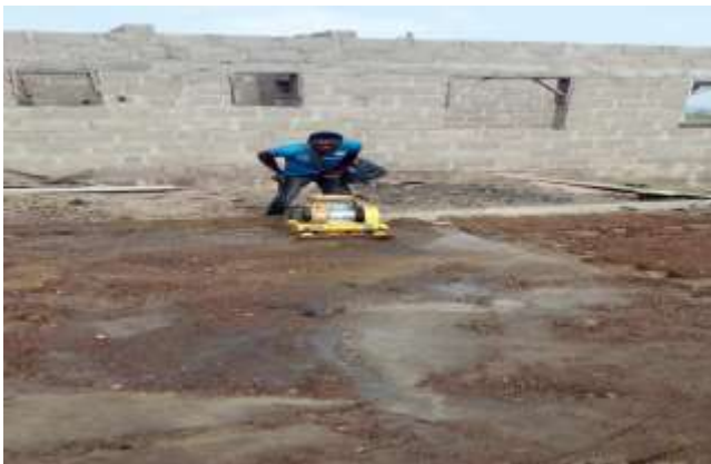
Image 6: showing compaction of soil by
