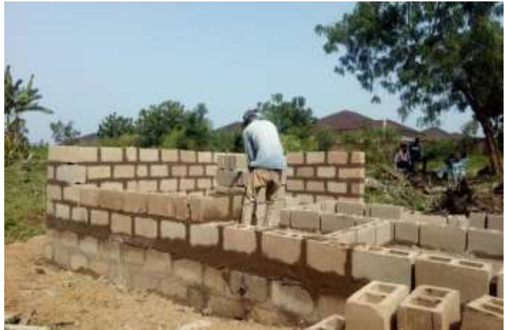
Image 9: showing block work in superstructure
