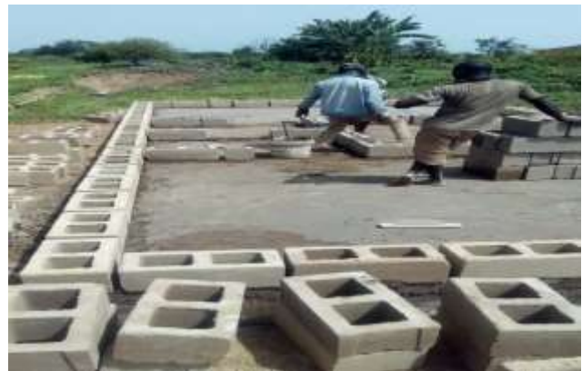
Image 9: showing block forming after DPC
