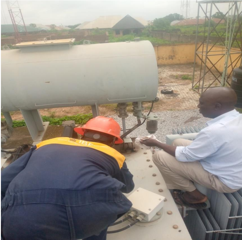
Checking the oil level at injection substation
