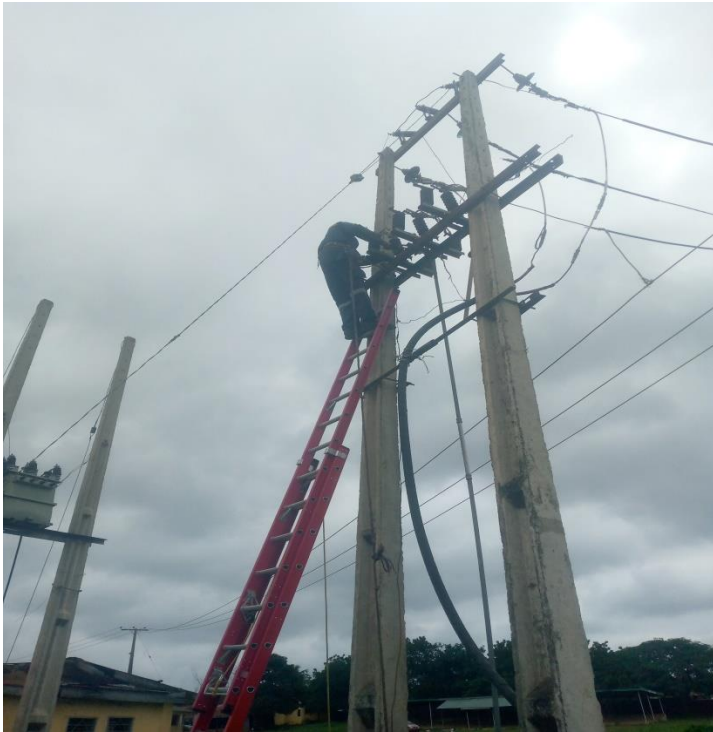
Replacement of silicon isolators with porcelain type isolators
