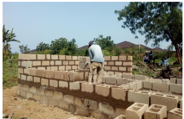
Image 9: showing block work in superstructure
